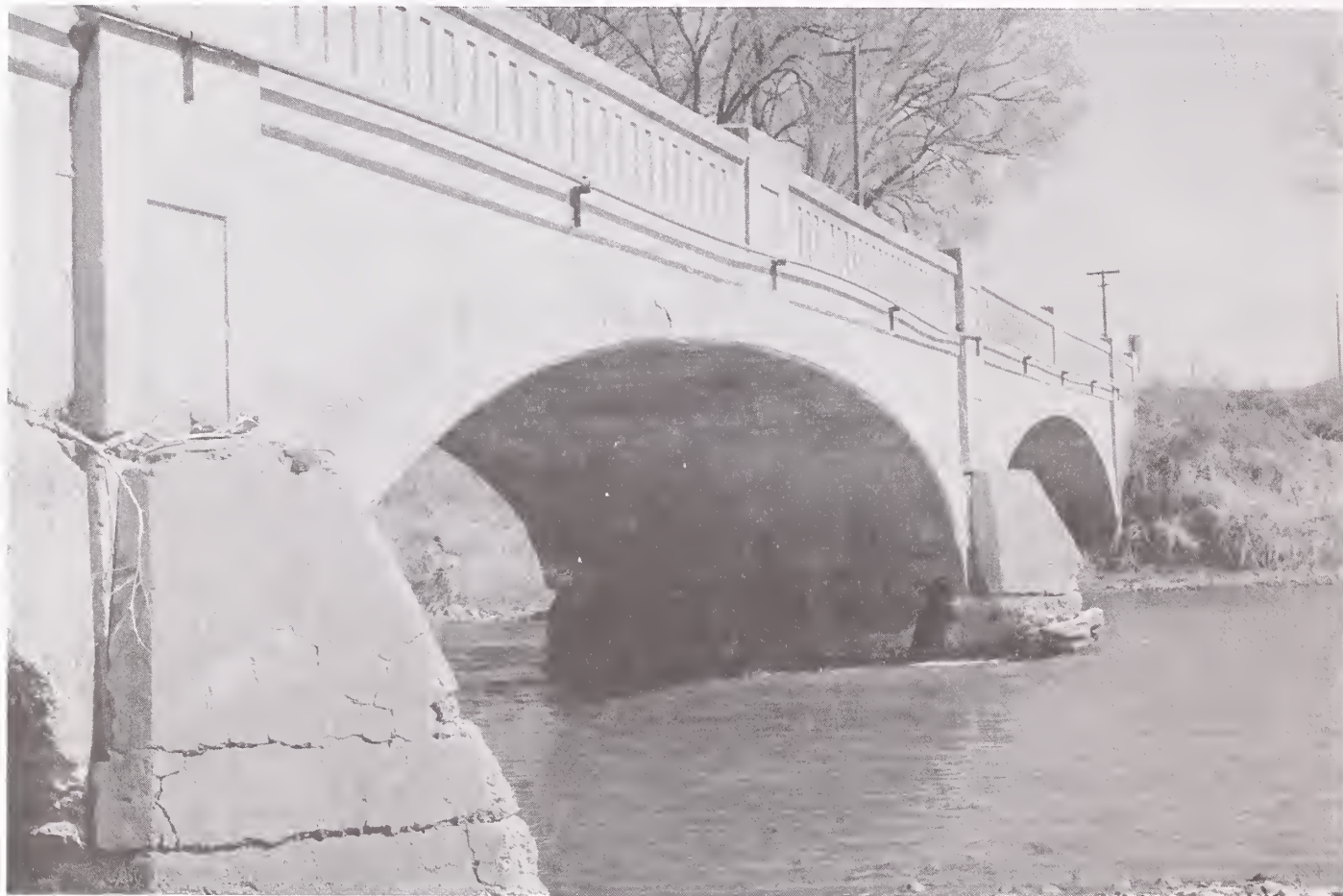
The Fromberg Bridge was the first large reinforced concrete bridge constructed in Montana.
